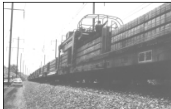
Amtrak's track laying machine, spreading the rails apart, removing wood ties, and inserting new concrete ties (above). A gantry crane (below) runs back and forth along the string of flat cars holding ties—delivering concrete ties to the TLM and removing wood ties from it.
