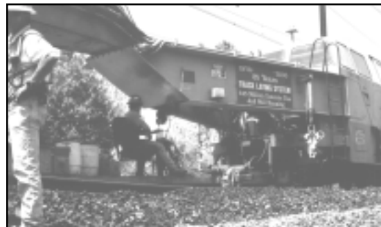
Amtrak's track laying machine, spreading the rails apart, removing wood ties, and inserting new concrete ties (above). A gantry crane (below) runs back and forth along the string of flat cars holding ties—delivering concrete ties to the TLM and removing wood ties from it.
